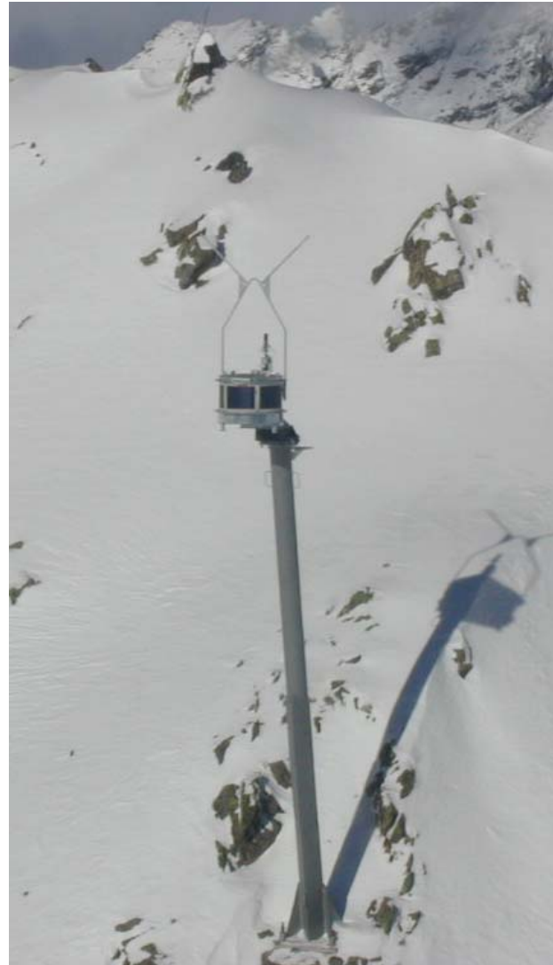
Figure 2: Wyssen Avalanche Tower installed in the big bowl of the Gonda avalanche.
